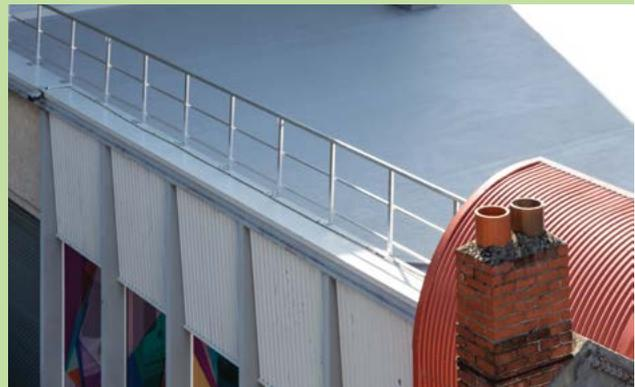
weldable Viking Enviroclad TPO membrane were installed with no end-laps as each roll extended the full width of the roof.
